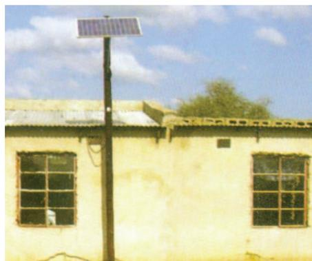
**Fig. 1** PV panels of typical solar system for domestic use in rural homes of Africa.
